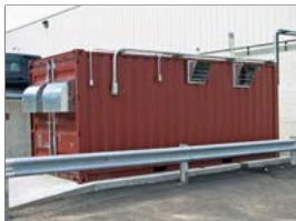
Stationary groundwater remediation system with 24 lbs/day ozone - turnkey package installed in 20' cargo container for air/ozone sparging at 80 injection wells, with PLC for user adjustable timing of pulsed sparging.
