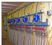
Stationary groundwater remediation system with 26 lbs/day ozone - turnkey package installed in 20' container for air/ozone sparging up to 8 CFM at 30 injection wells, with PLC for user adjustable timing of pulsed sparging.
