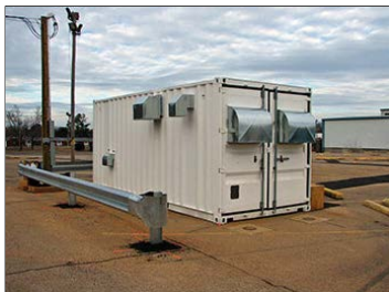
Stationary groundwater remediation system with 26 lbs/day ozone - turnkey package installed in 20' container for air/ozone sparging up to 8 CFM at 30 injection wells, with PLC for user adjustable timing of pulsed sparging.
