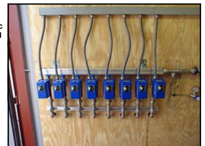
PLC Control Panel (sparge time controller)
