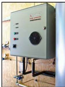
Ozone Generator (24 lbs/day water cooled)
