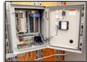
PLC for controlling 12 banks of sparging manifolds and ozone
