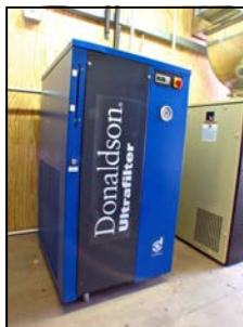
Water Chiller (ozone generator cooler)
