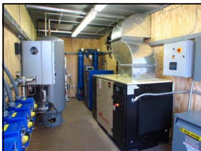
Ozone Generator (24 lbs/day water cooled)
