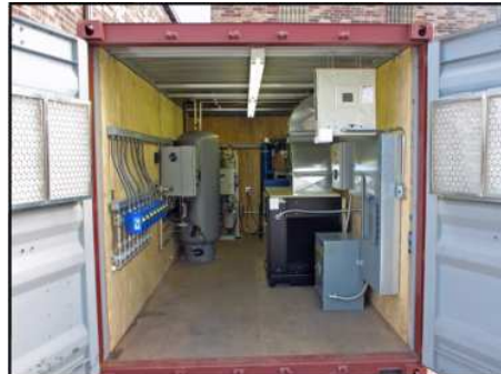
Banks of Sparging Manifolds (with sparge lines connected)
