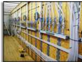
Banks of Sparging Manifolds (with sparge lines connected)
